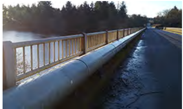
Water Main Crossing Bridge QIN Planning
