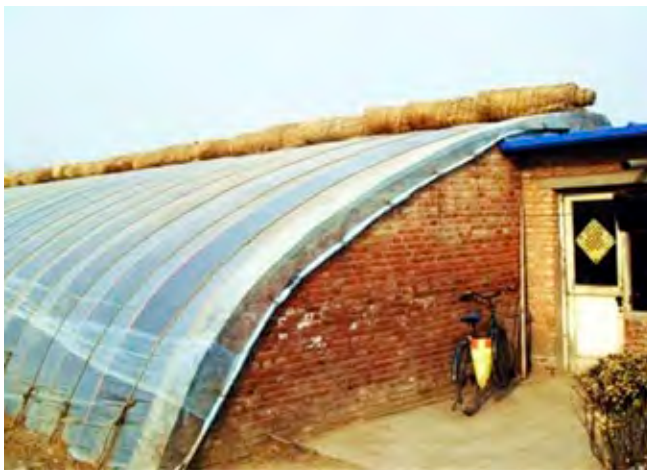
Figure 2. Chinese Solar Greenhouse (De Decker, 2015)
