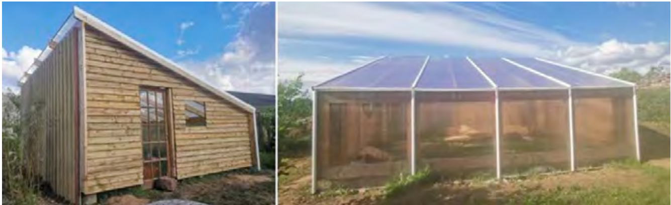
Figure 1. Passive solar greenhouse (Crook, 2021)
